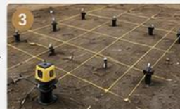
Mark Footing Points Use grid or laser to mark all footing or pier locations.
