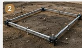
Connect Rails Adjust rails to dimension and lock in place.
