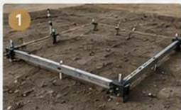
Set Corners Position and lock corner brackets. Square is set.
