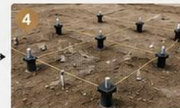
Install Footings/Piers Set to required height. Check level.
