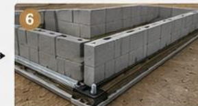
Lay First Row Apply mortar and lay first row using locators.
