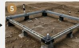
Install Starter Tracks Level and lock starter tracks in place.
